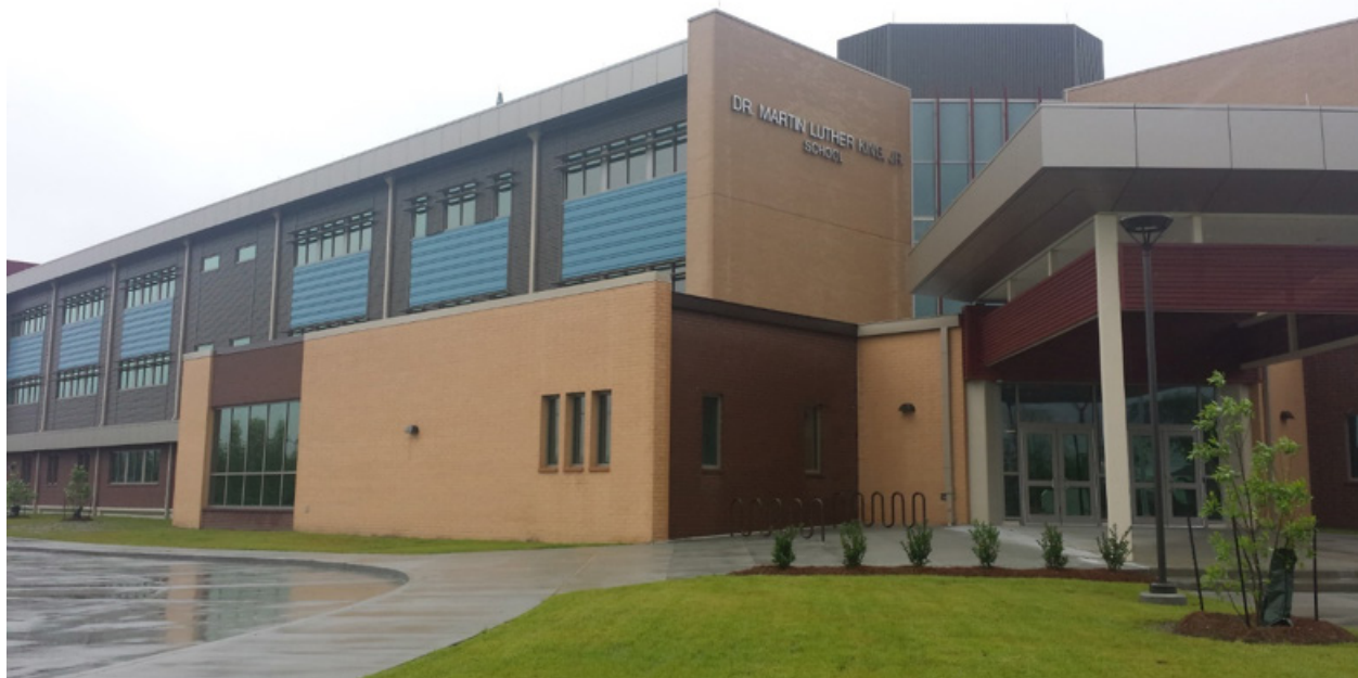
The newly built Martin Luther King High School in Lower 9th Ward on former site of Alfred Lawless High School (Photo Credit: Kristen Buras, 2016)
